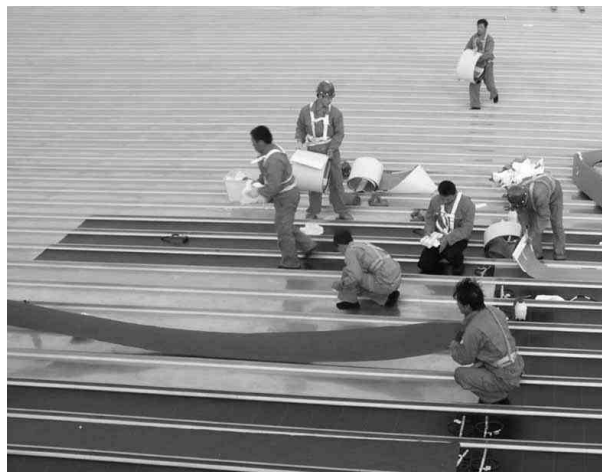
Fig. 3. The Uni-Solar a-Si factory produces peel-and-stick thin-film PV roofing material. The product's easy installation is demonstrated on a building in China.
