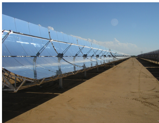
Fig. 1. New APS solar power plant using Solargenix parabolic trough concentrator and Schott receiver
