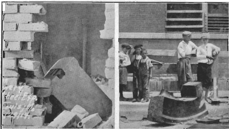
FLY-WHEEL EXPLOSION UNION BREWING CO., ST. LOUIS, MO., 40,000- POUND WHEEL ON ICE MACHINE RUNNING NORMALLY AT ONLY 50 R.P.M. MACHINE RACED AND BURST WHEEL BY CEN- TRIFUGAL FORCE, HURLING 8,000-POUND CHUNKS GREAT DISTANCES. RIM SECTION WAS 13"x16", TO BREAK WHICH REQUIRED 4,000,000 POUNDS. LOSS $13,423. WHEEL INSURED.
