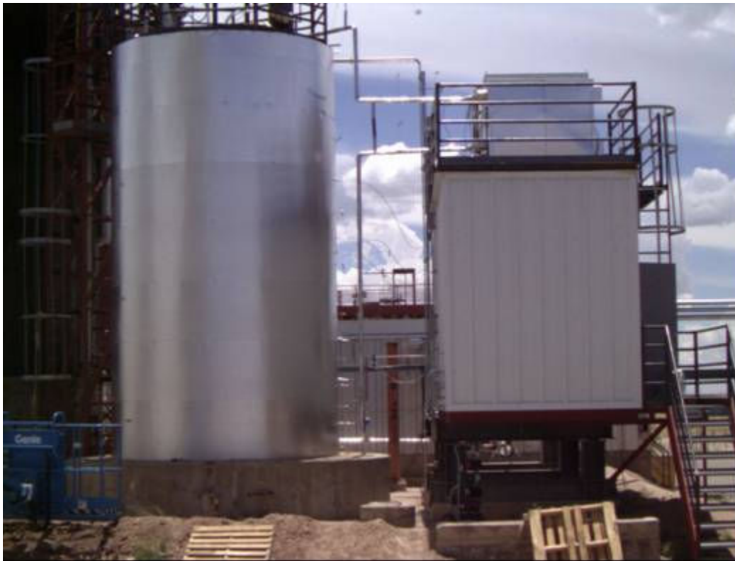
The above photo shows the thermocline tank fully heat traced, and the initial layers of insulation applied. The image below shows the completion of insulation, as well as the cooler on the right.
