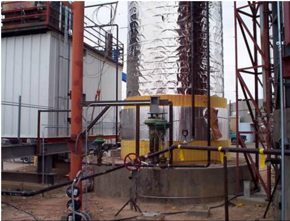
The above photo shows the thermocline tank fully heat traced, and the initial layers of insulation applied. The image below shows the completion of insulation, as well as the cooler on the right.
