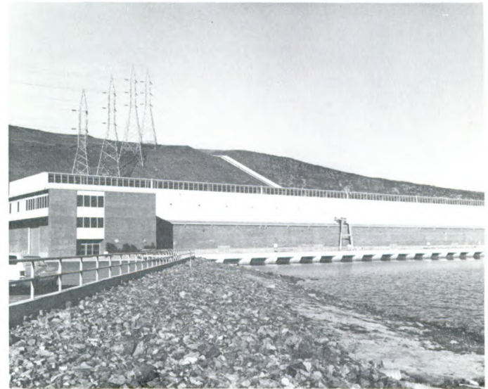
San Luis Pumping-Generating Plant
