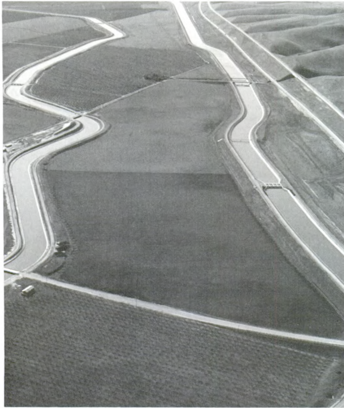
Delta-Mendota Canal and California Aqueduct
