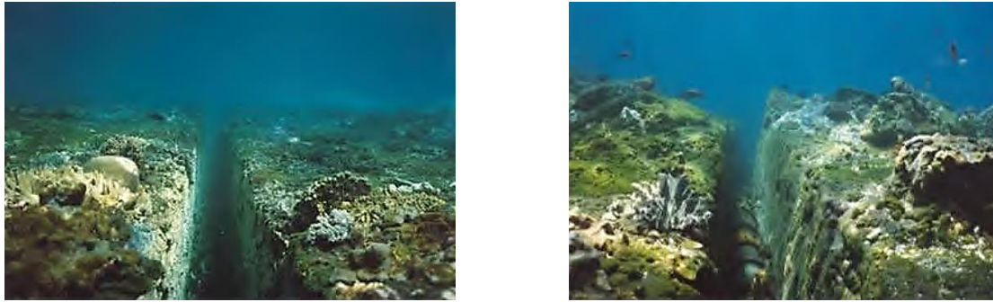
Fig. 31 – The trench of a submarine power cable
