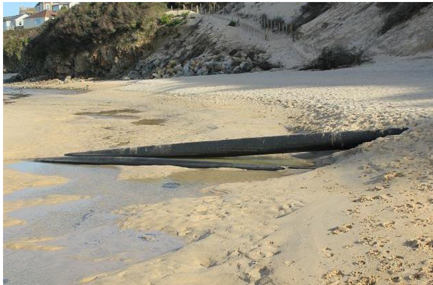
Fig. 17 – Cable exposure due to waves' action on a sandy beach in Great Britain (Source: aphotomarine.com )
