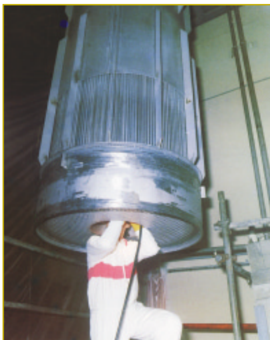
Repairing a washed and decontaminated intermediate heat exchanger
