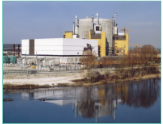
The Creys-Malville plant
