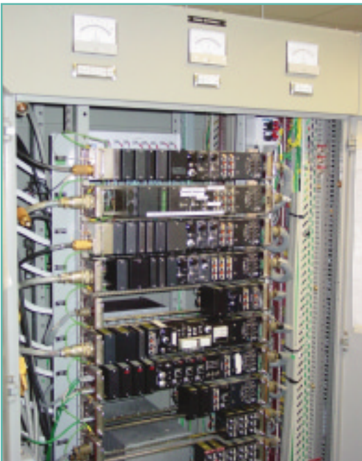
Neutron chambers' electronic cabinets
