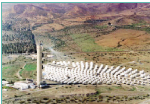
Almeria solar power plant
