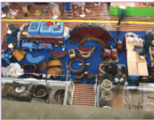
Turbine undergoing overhaul
