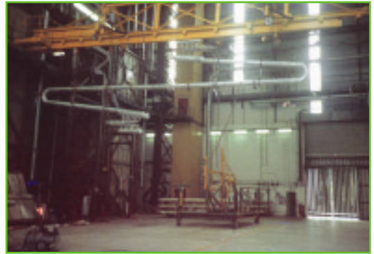
Steam generator module during handling
