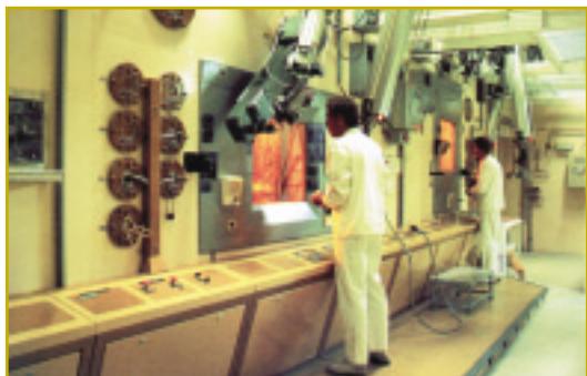
Spent sub-assembly dismantling cell
