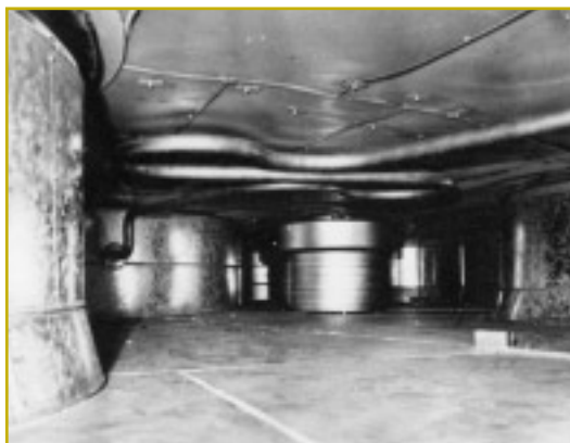
Space between roof and slab of the reactor
