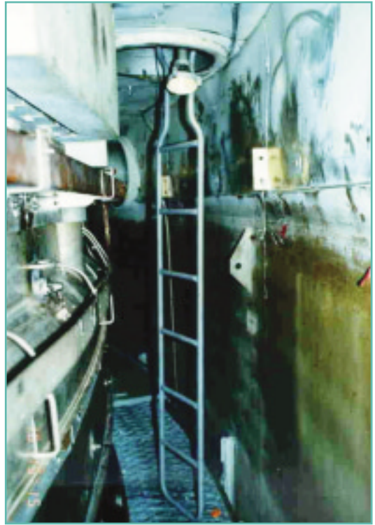
Space between main vessel and containment vessel
