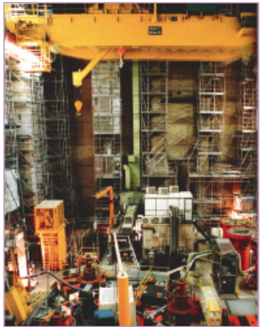
Hall of the reactor building during seismic reinforcement work
