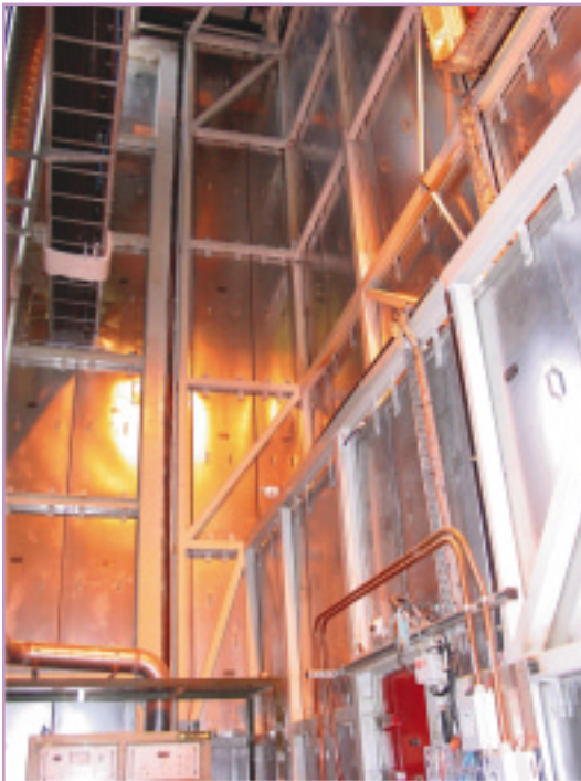
Steam generator building partitioning
