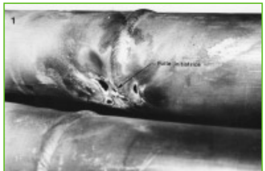
Steam generator tube with leak
