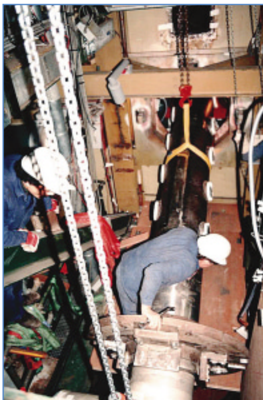
Replacing secondary cooling circuit pipes
