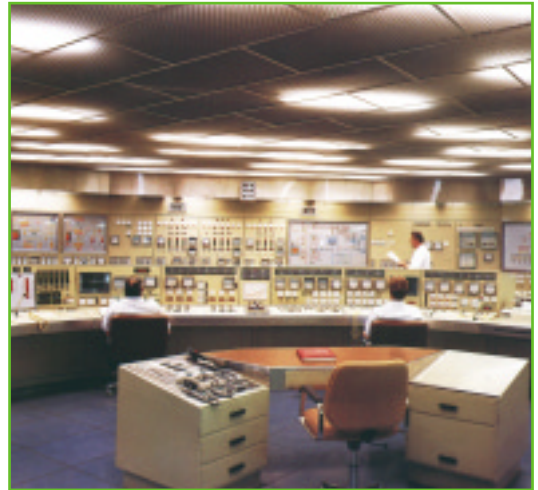
The control room
