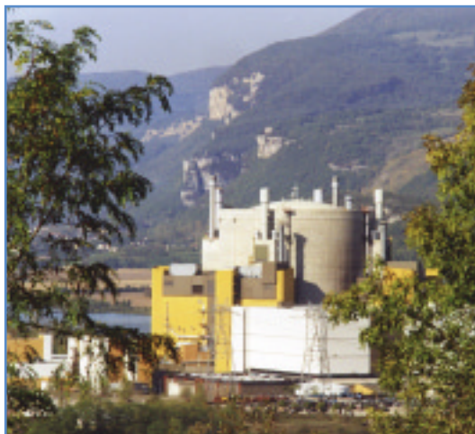
The Creys-Malville plant
