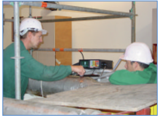
Inspecting secondary cooling circuit pipes
