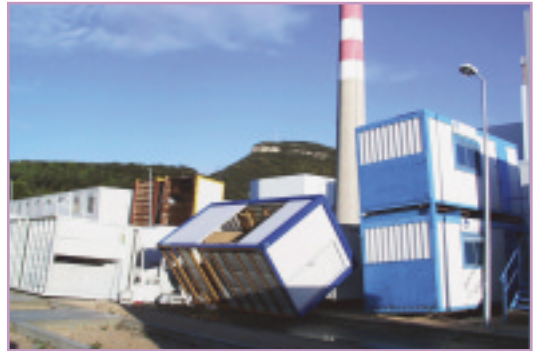
Sub-contractors reception area following the mini-tornado of September 1999
