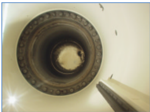
The primary sodium seen through a slab penetration
