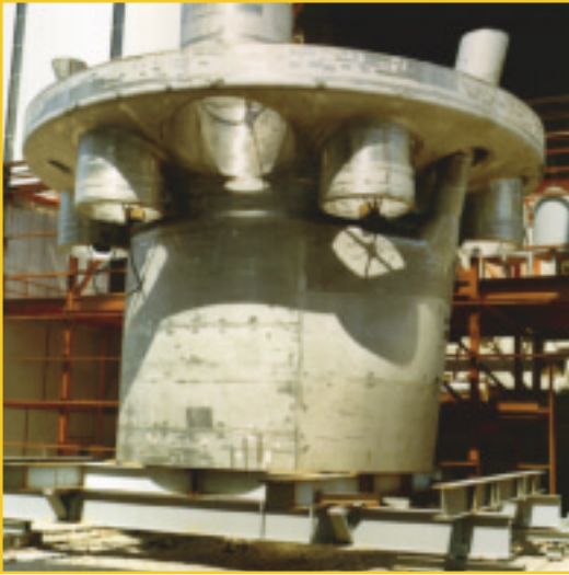
Installing the primary vessel
