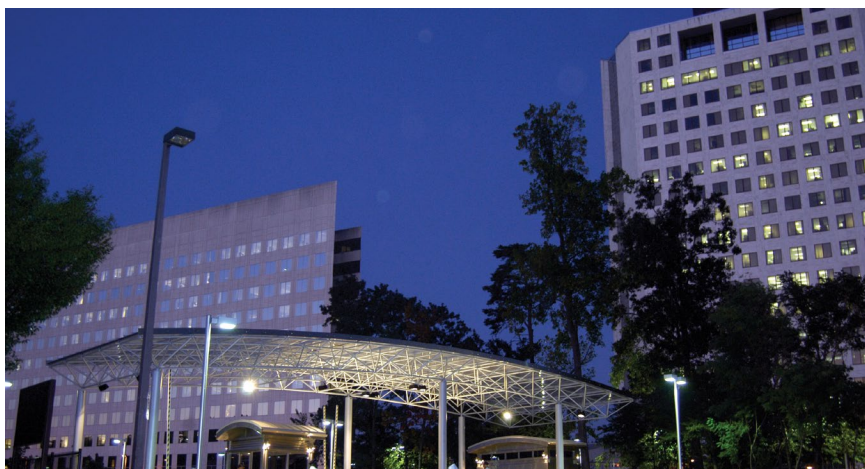
The NRC Headquarters complex is located in Rockville, MD.
