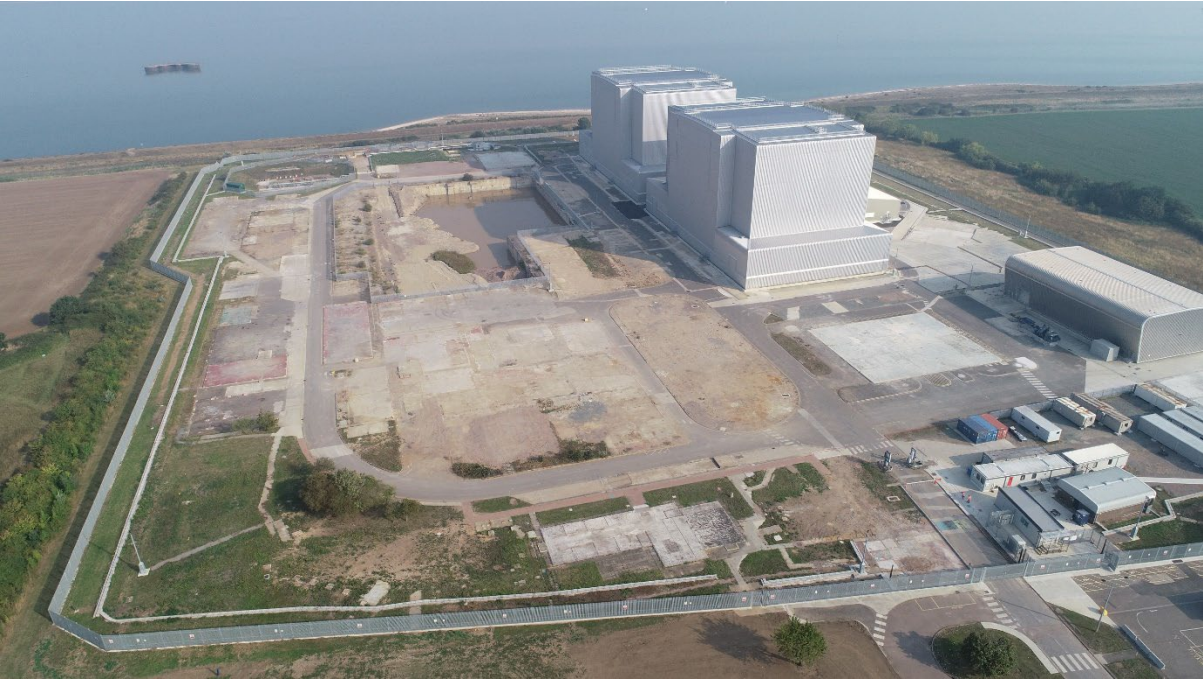
Bradwell Magnox station in its interim end state
