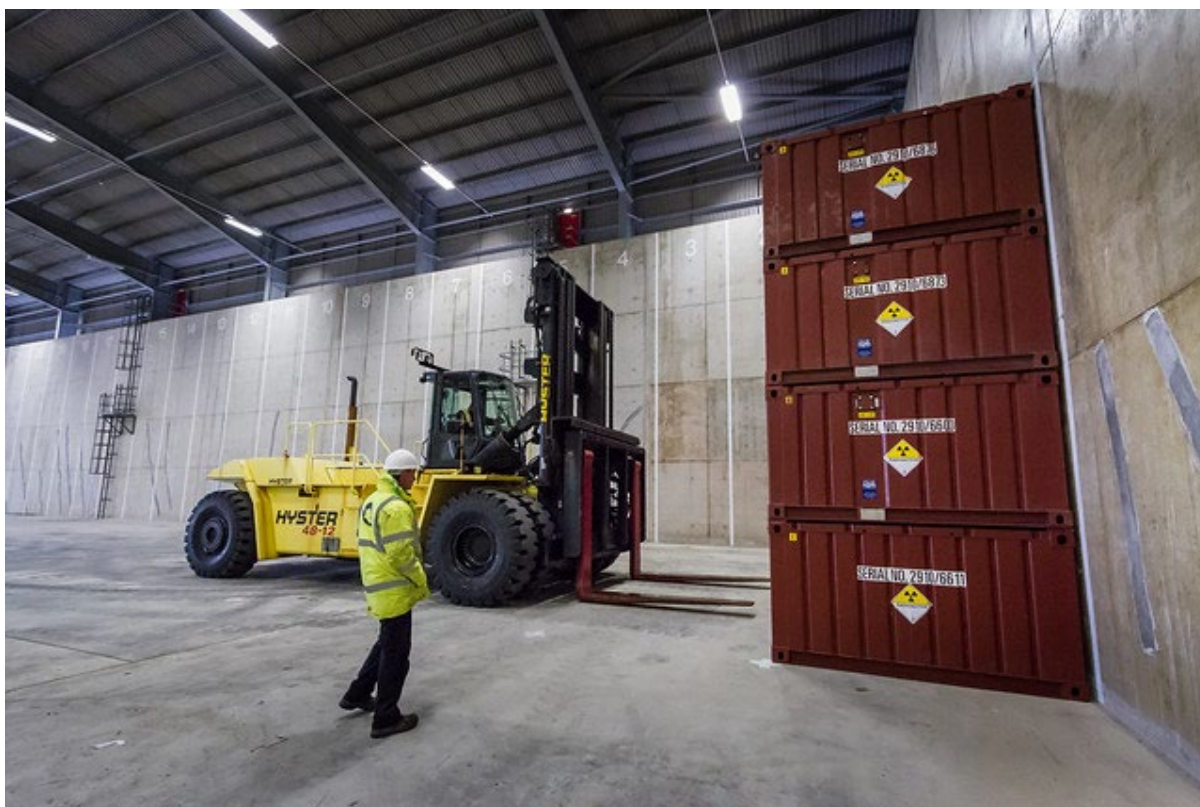
Inside the Dounreay LLW facility
