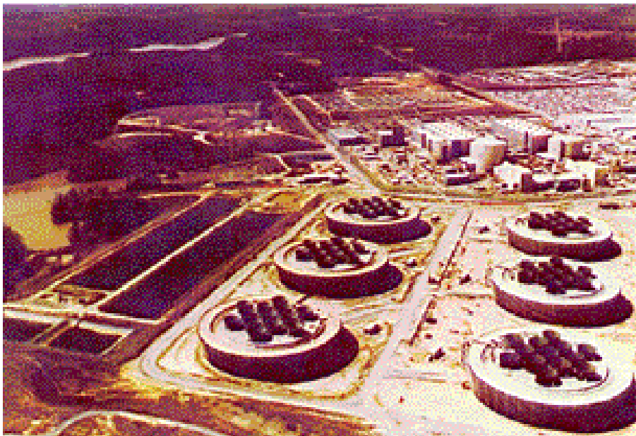
Figure 1. Catawba Nuclear Station.
