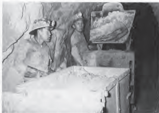
Miner Alfred Francis operating a mucking machine. Bill Shorty, a train operator is in the foreground. Taken at the Rico mine in Colorado. Photograph by Ralph Leubben, 1953.
