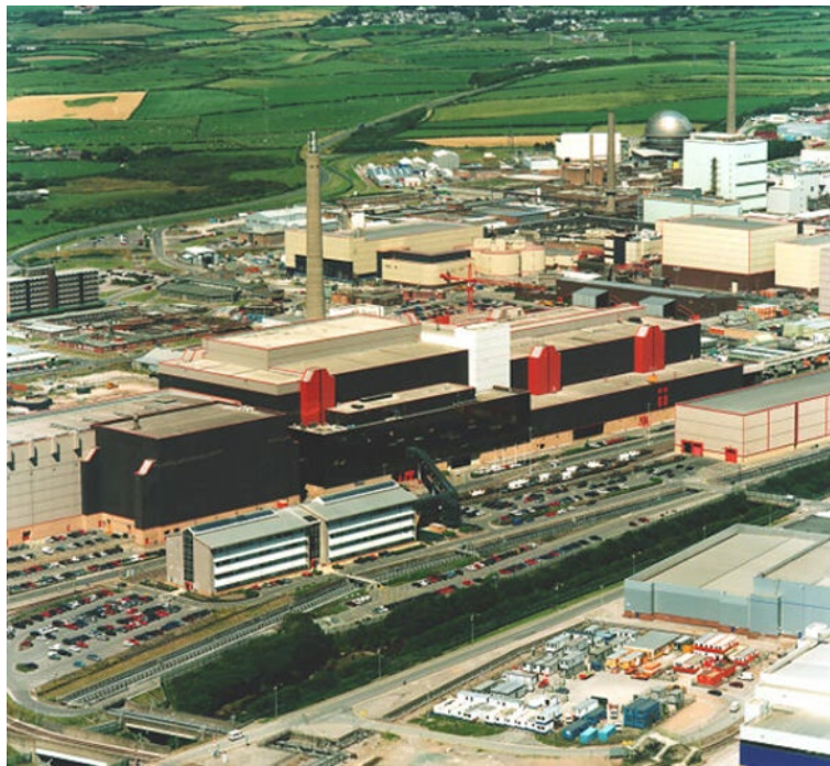
Figure F1-3. Sellafield site, U.K., with THORP and B205 reprocessing plants (BNFL, plc).
