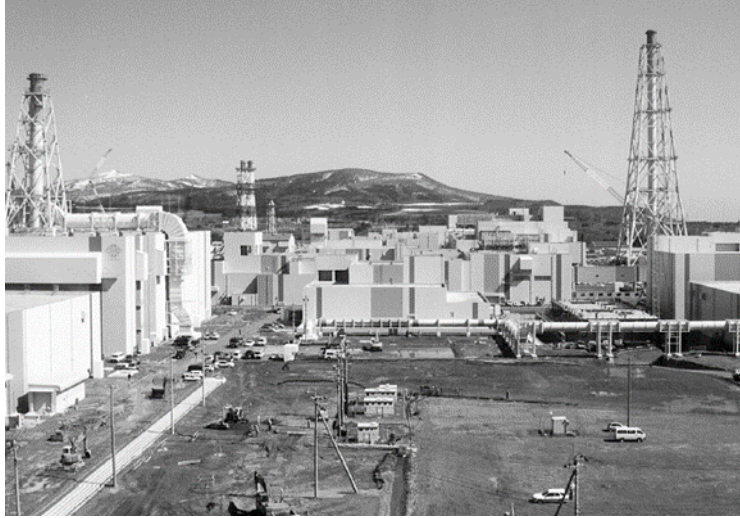
Figure F1-4. Rokkasho-Mura site, Japan, with Rokkasho Reprocessing Plant (JNFL).
