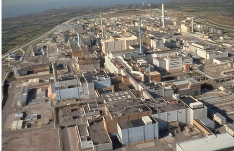
Figure F1-2. La Hague site, France, with reprocessing plants, UP2-800 and UP-3 (AREVA).
