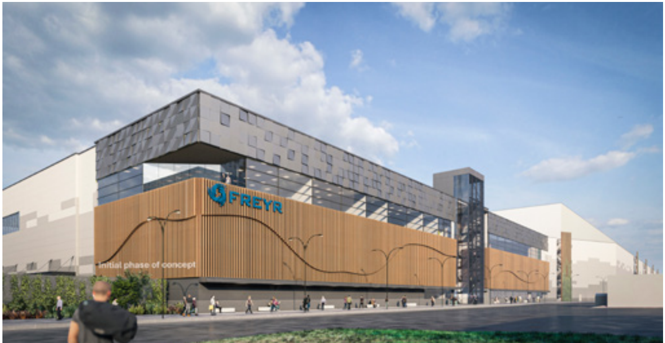
Initial view of FREYR’s Giga Arctic Factory in Mo i Rana, Northern Norway. Production is due to start in the first half of 2024. Image, courtesy FREYR Battery.
