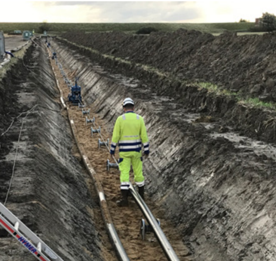
Installation of the NordLink cable in Germany. Image courtesy NKT.
