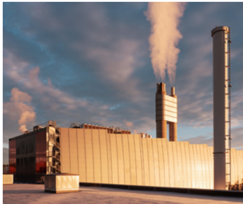
The waste-to-energy plant at Klemetsrud in Oslo is implementing CCS technology to capture up to 400,000 tonnes of CO 2 each year from 2026. More information about the project and technology can be found here . Image courtesy of Fortum Oslo Varme AS
