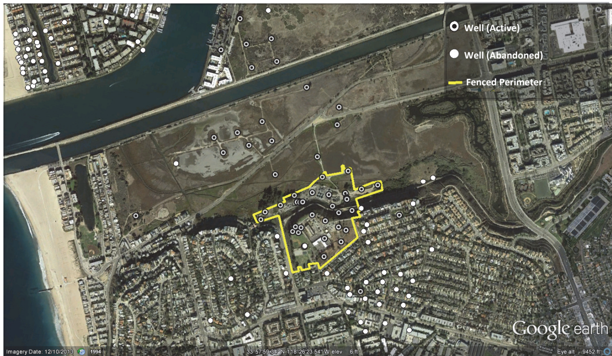
5 Figure PEB-3 6 Southern California Gas Company 7 Aerial View of Playa Del Rey Underground Storage Field
