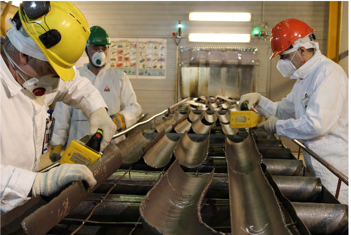
FIG. 2. Workers dismantling the turbine hall at Ignalina nuclear power plant measure scrap metal for traces of radiation (file photograph).
