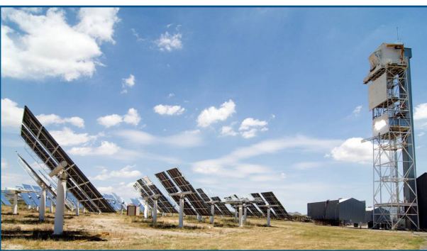
The thermochemical solar hydrogen plant at Plataforma Solar de Almeria, Spain, with the solar tower where the scaled-up HYDROSOL-II reactor is installed
