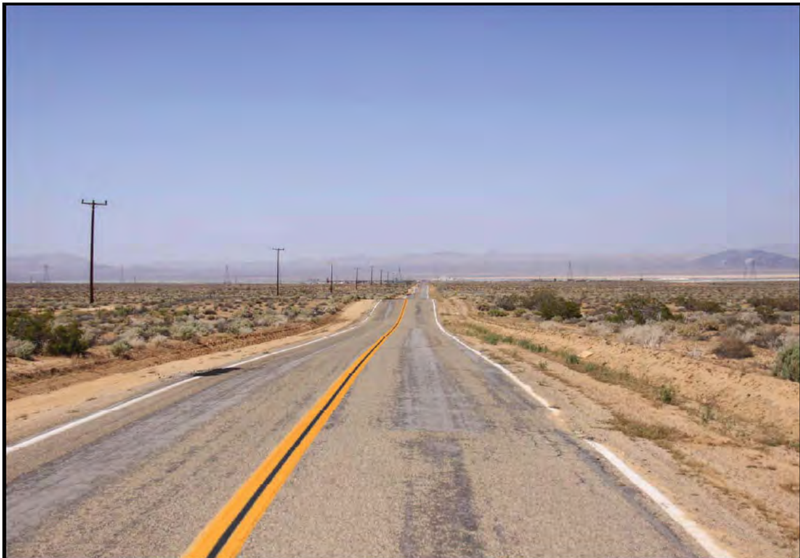
KOP 1 – View From Harper Lake Road near Phoenix Road - Post Project
