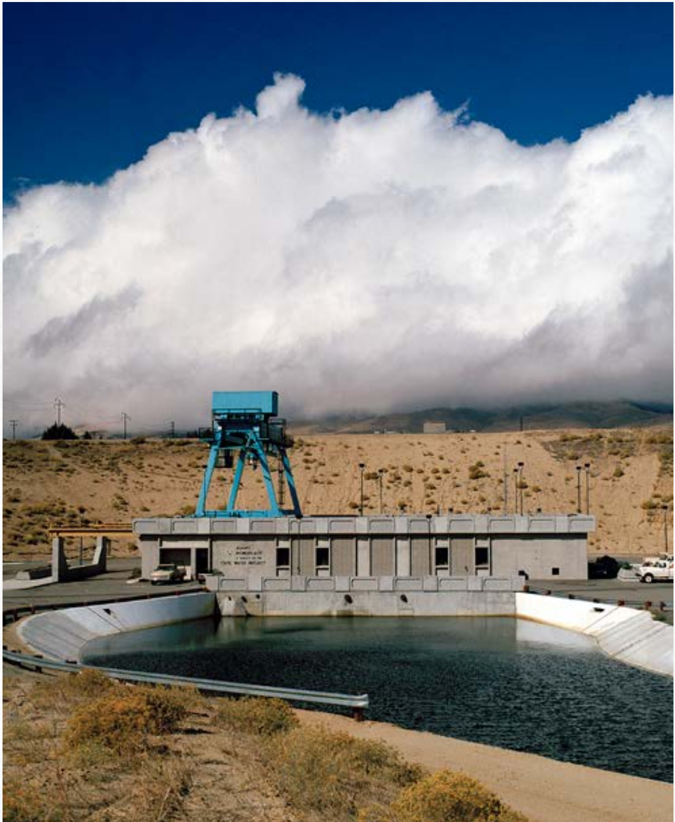
Alamo Powerplant completed in 1985 on the East Branch of the State Water Project has a generating capacity of 15 megawatts.
