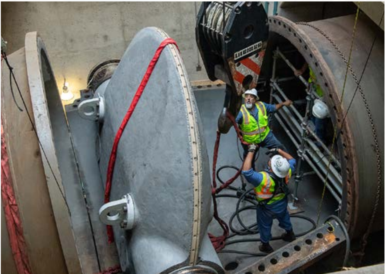
Valve refurbishment at Gianelli Pumping-Generating Plant in Gustine, California.
