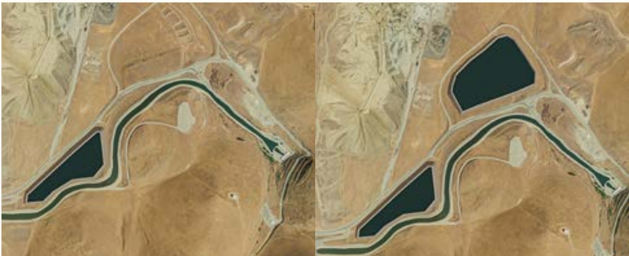
Conceptual renderings of potential off-stream storage locations near Edmonston Pumping Plant in Kern County.
