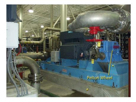
Figure 3 - Tampa Bay Desalination Plant Pelton Wheel Energy Recovery System
