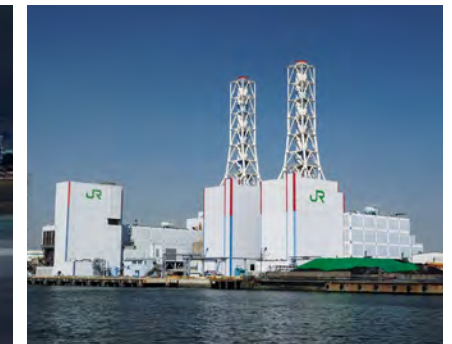
Kawasaki Thermal Power Station
