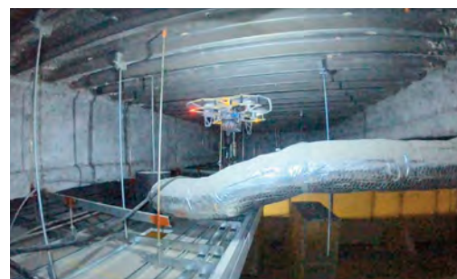
For inaccessible areas of sites, we use small drones specially designed for restricted spaces to acquire images and point cloud data.
