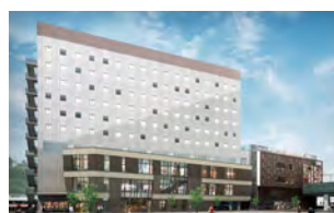
Iwaki Station South Entrance exterior
