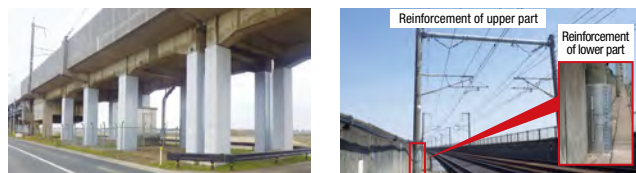
Seismic reinforcement of elevated railway tracks
