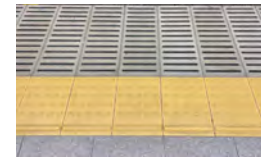
Braille blocks that indicate which direction is away from the edge of the platform
