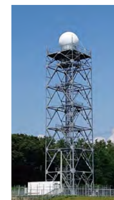
Doppler radar installed at Kurumori, Sakata
