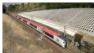
Cutting slope protection (spray framework)
