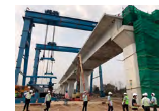
Viaduct construction site (courtesy of JICA*)
