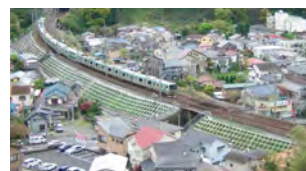
Embankment slope protection (spray framework)
