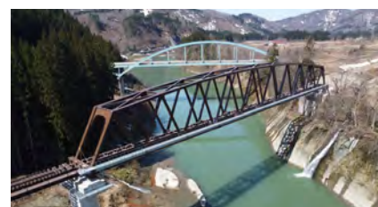
Tadami Line restoration work (No. 7 Tadami River Bridge)
