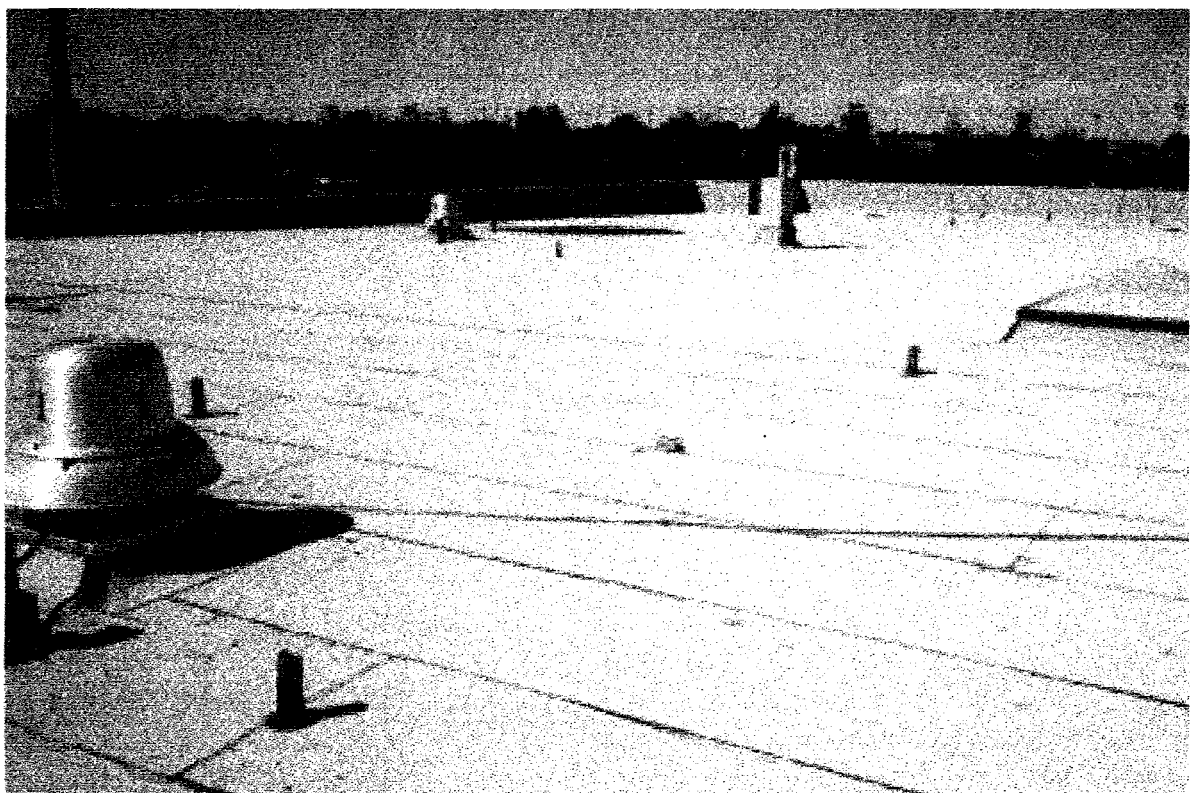
Figure 2.2 Rooftop of the Kaiser Permanente Medical Office Building in Davis, California, light gray capsheet with solar reflectance of 0.24.
