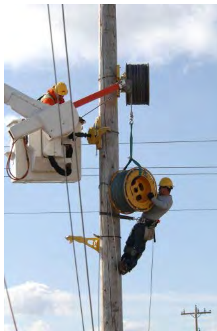
Idaho Power linemen install upgrades.
