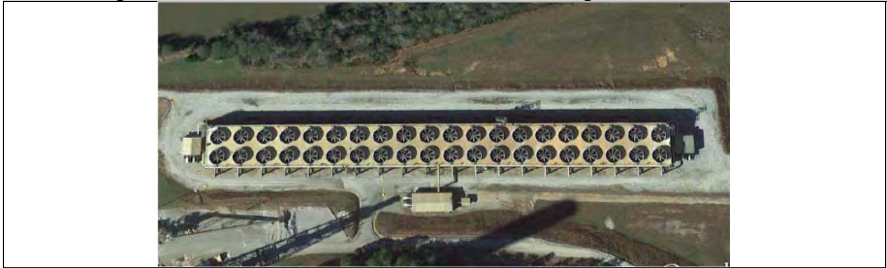
Figure 9b. Plant Yates 40-Cell Back-to-Back Cooling Tower – Plan View 65
