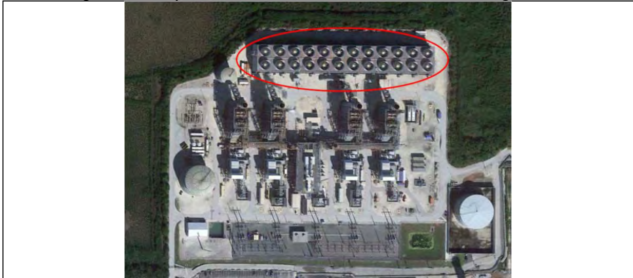
Figure 3. Turkey Point Unit 5 24-Cell, Back-to-Back Wet Cooling Tower 28
