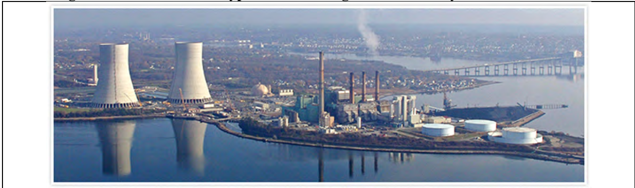
Figure 6. Natural Draft Hyperbolic Cooling Towers at Brayton Point Station 46
