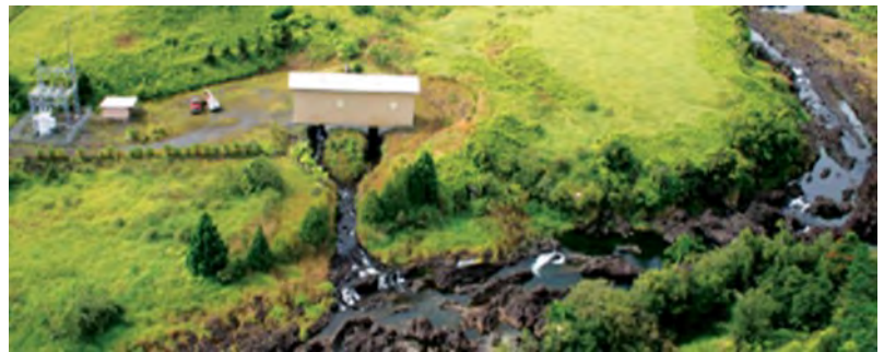
Wailuku River Hydroelectric Power Plant, 11 MW, Hilo, Hawaii
