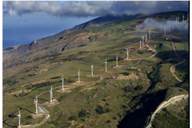
Kaheawa Wind Power I, 30 MW, Maui
