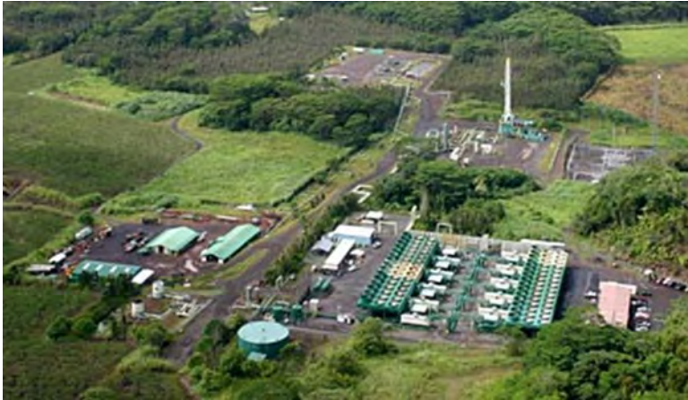
Puna Geothermal Venture Power Plant, Pahoehoe, Hawaii Island
