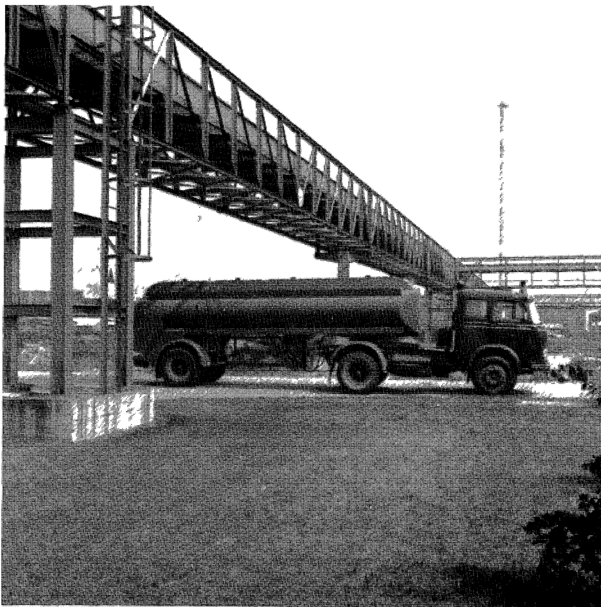
FIG. 1. Tanker truck and pipe hanger gallery for the transport of low level liquid wastes
