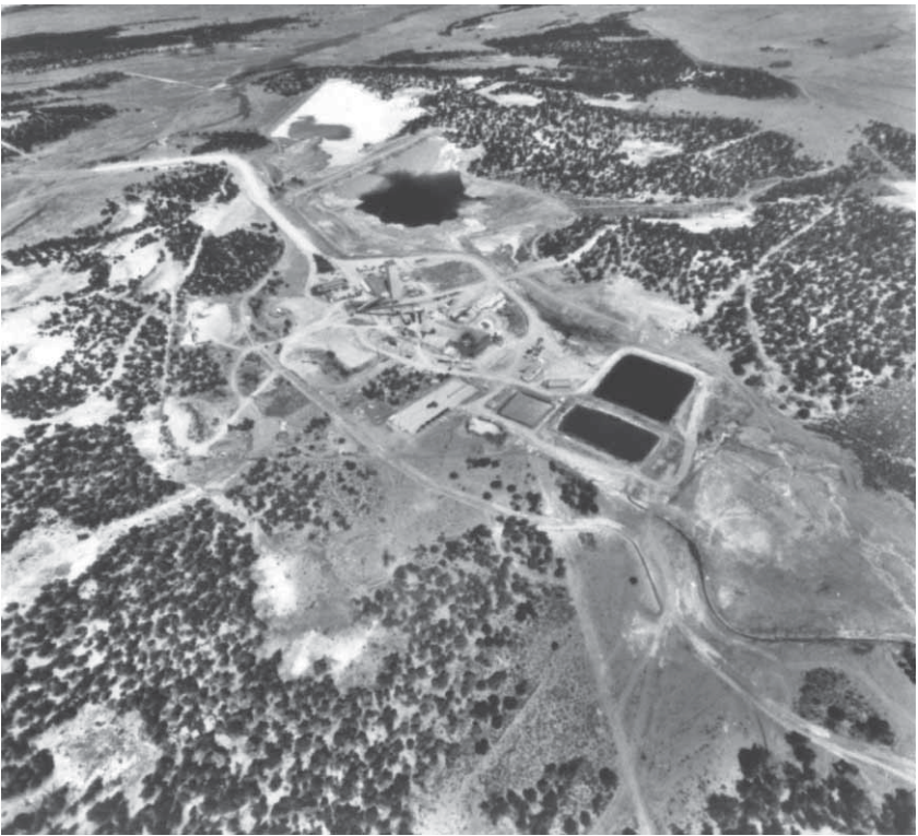
The Rio Algom uranium mill and tailings site in Utah is undergoing reclamation.
