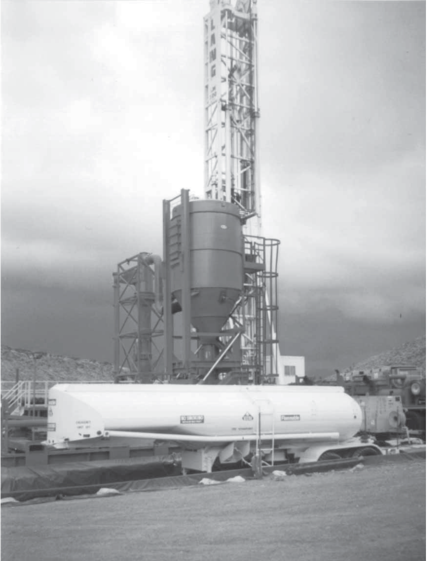
LM-300 drill rig at Yucca Mountain, Nevada, obtained underground rock and soil samples that scientists examined to help determine site suitability for high-level waste disposal.
