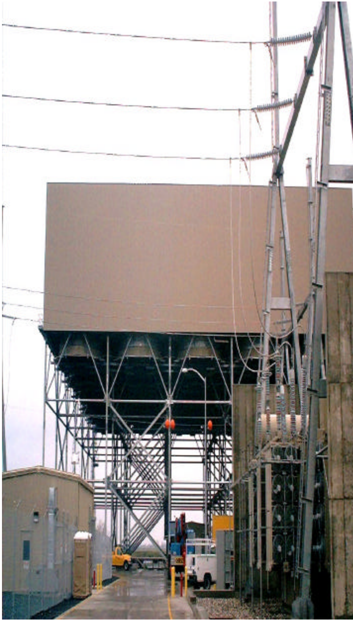
Figure C-10 ACC at Sutter Energy Center
