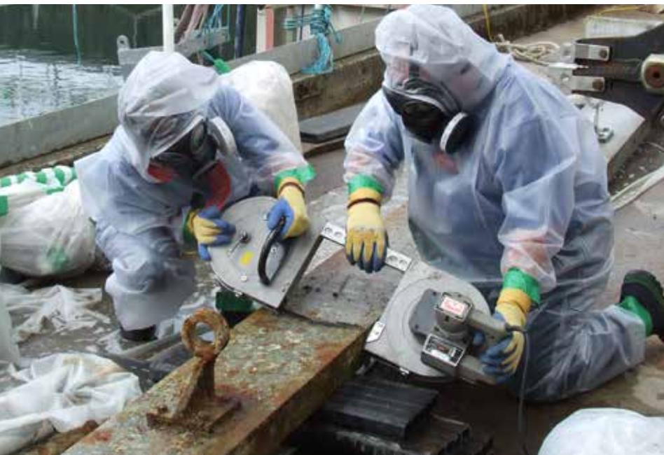
**Decommissioning staff cutting down a piece of large metal equipment at a nuclear facility.**
