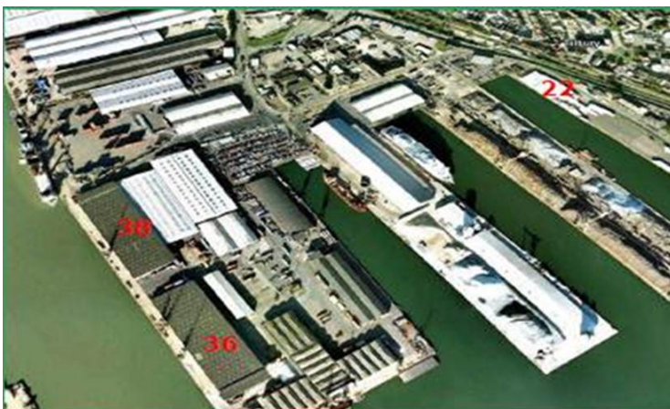
Figure 12: Aerial image of the Riverside Resource Recovery Ltd's Crane at berth 22 and the Ballast Phoenix IBA processing site, berths 36/38.
