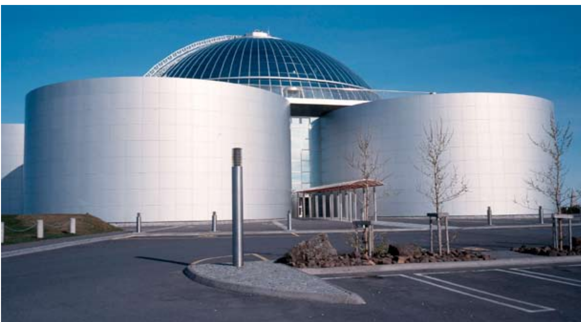
Geothermal water tanks, with restaurant Perlan on top.
