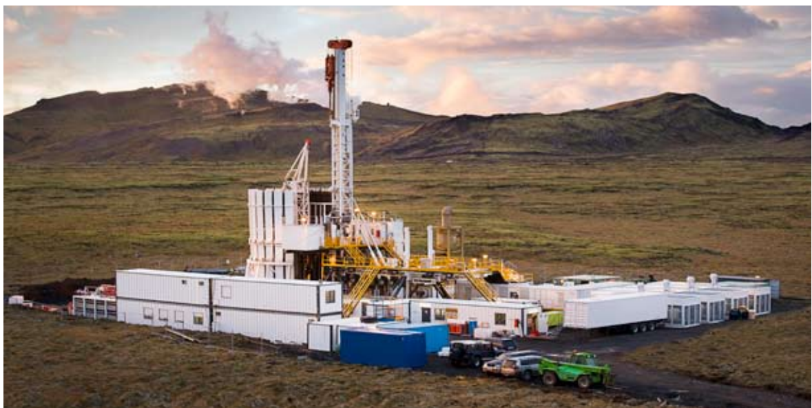
A drilling rig at Hellisheidi.
