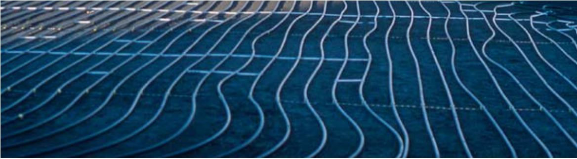
A snow-melting system being installed.
