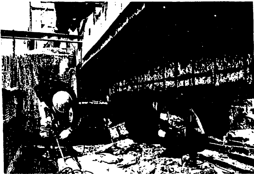
REMOVAL OF DETERIORATED CONCRETE
