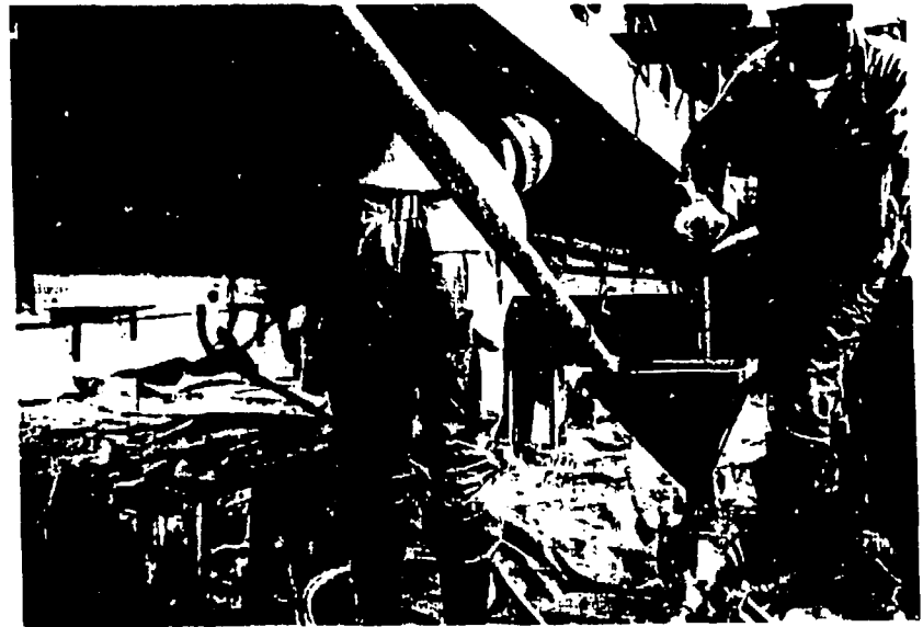
GROUTING OF POLYMER CEMENT MORTAR INTO PREPLACED AGGREGATE
