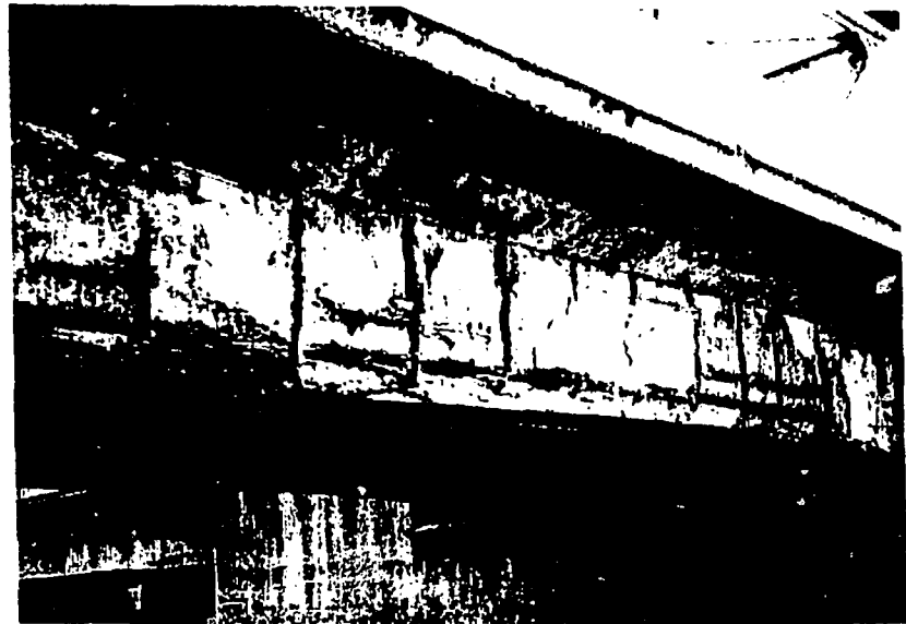
CORROSION OF STEEL REINFORCEMENT
