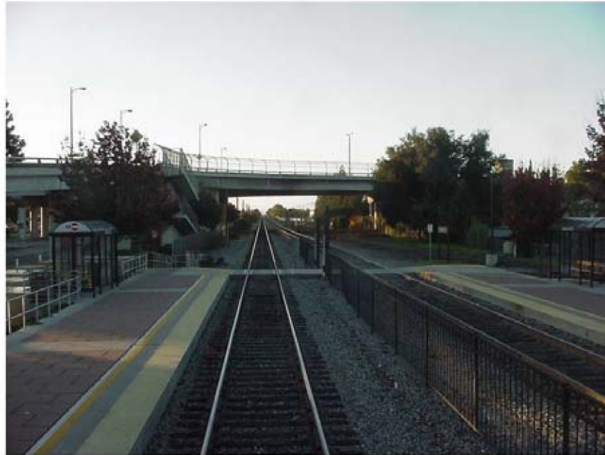
PEDESTRIAN WALKWAY WITH OVERBRIDGE PROTECTION BARRIER
