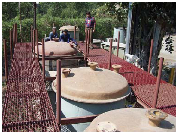
Figure 8. Pilot plant facility (under construction) for uranium recovery from seawater (27).
