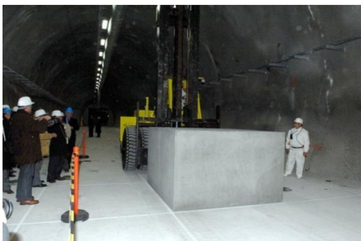
*FIG. A-13. Emplacement of the first waste disposal package at the disposal facility in Bataapáti, Hungary.*
