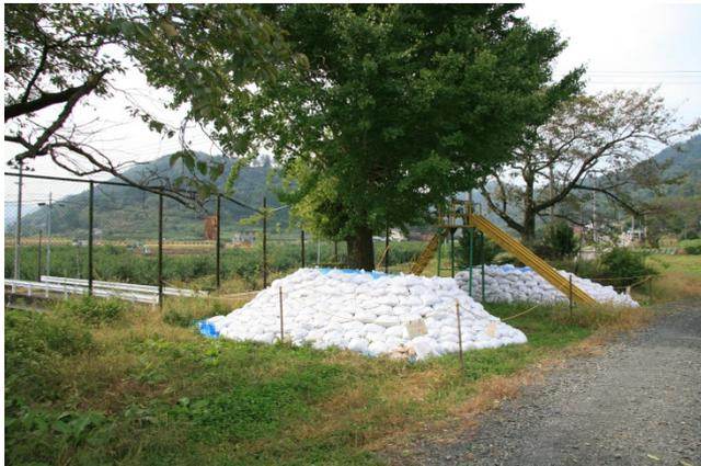
*FIG. A-16. Temporary storage of soil removed at a model remediation project at the Tominari elementary school, city of Date, October 2011.*
