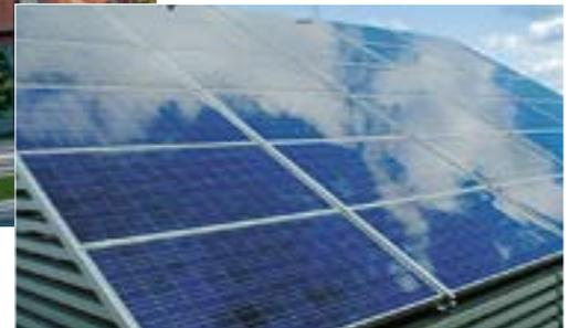
**Solar cells.** The sun's luminous energy is captured and converted into electrical energy in solar cells. The energy from a 1m<sup>2</sup> solar cell module produces approximately 100 kWh/year, which corresponds to the domestic electricity requirements of 3m<sup>2</sup> residential floor space.
