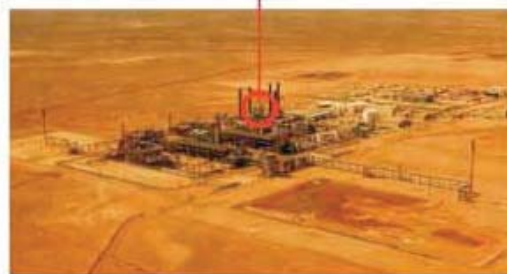
At In Salah, Algeria, natural gas purification by CO 2 removal plus CO 2 pressurization for nearby injection
